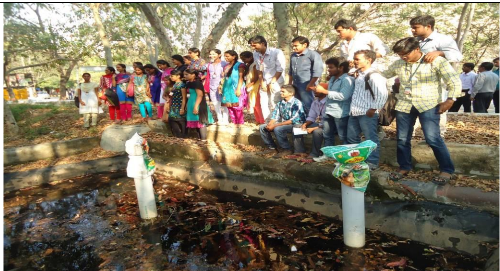
CMR engineering collegestudents visiting the rainwater harvesting systems in the campus
